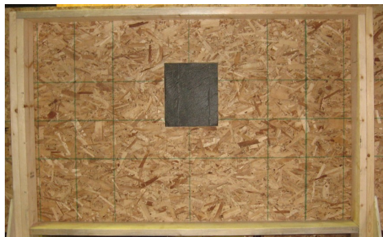
Frame opening and cut out hole for the termination and thimble as shown in fig. #6
